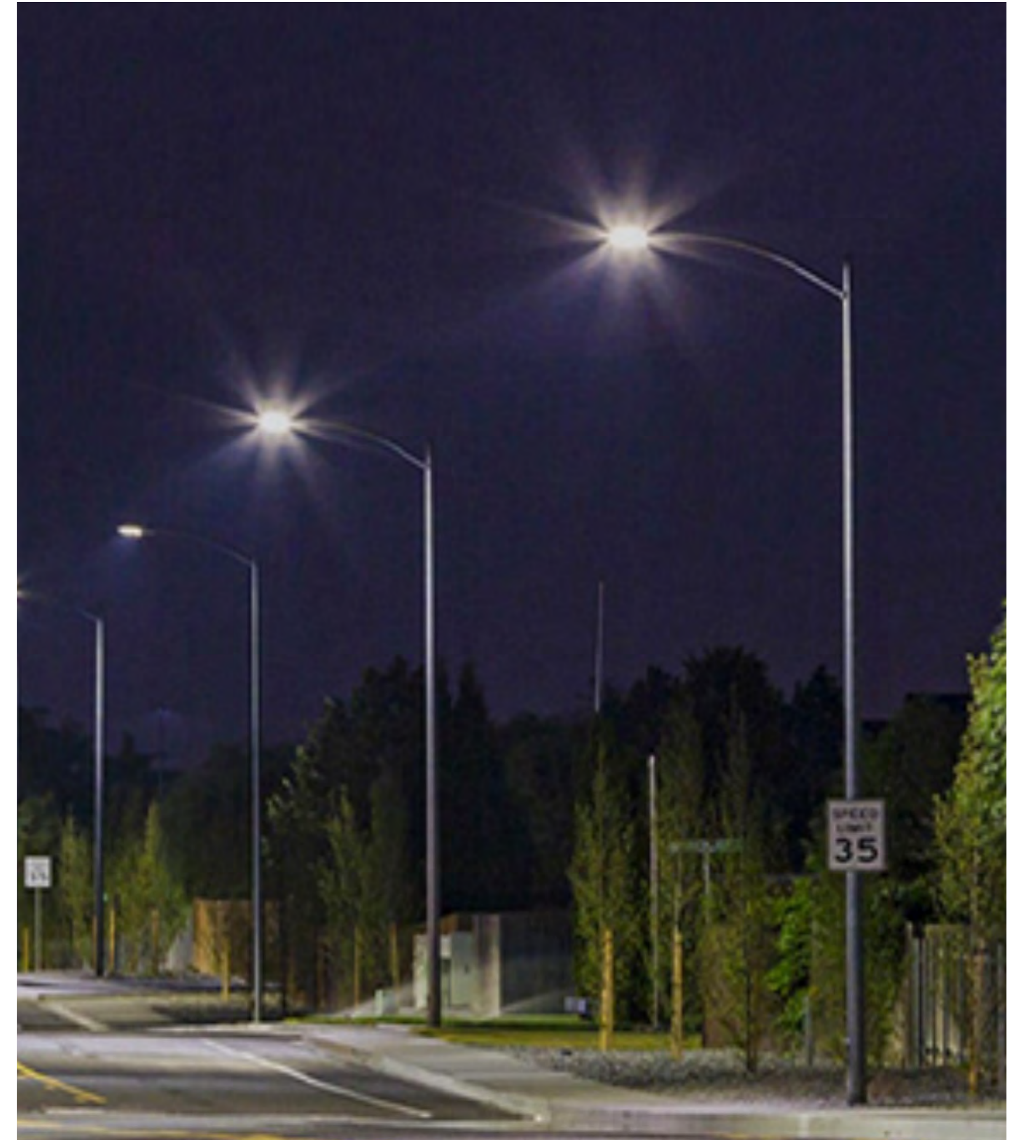
MNDOT COBRA LIGHTING
